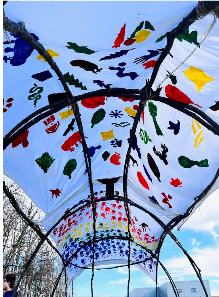
Student artwork freshly installed on the frame, to be covered with canvas.
