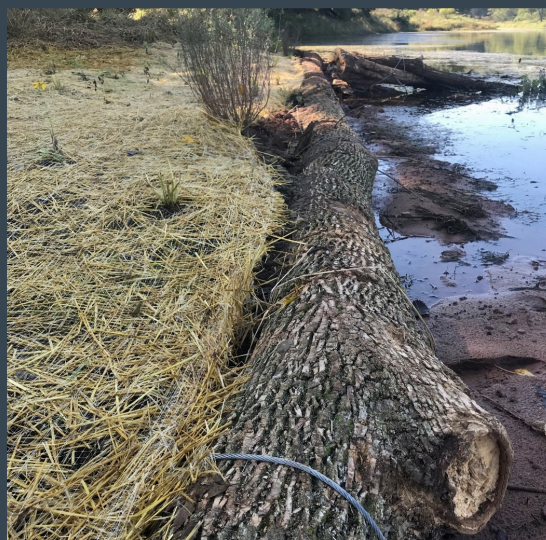
Dutch Hollow Shoreline Stabilization Project using log revetments, fish sticks, and native plants
